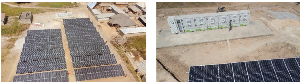
FIGURE 5.5: Solar Hybrid Mini Grid with Containerized Energy Storage Solutions Installed by PowerGen in Dancitagi, Nigeria
