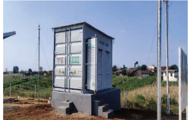
FIGURE 5.6: Solar Mini Grid with Containerized Battery Energy Storage System in Makhala, India
